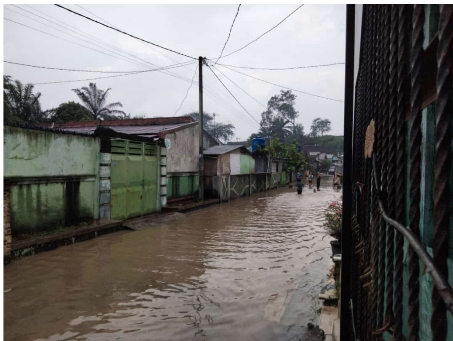
Figure 1. Flooding that occurred on Jalan Marga Anak Tuha, Rajabasa District, Bandar Lampung City.
