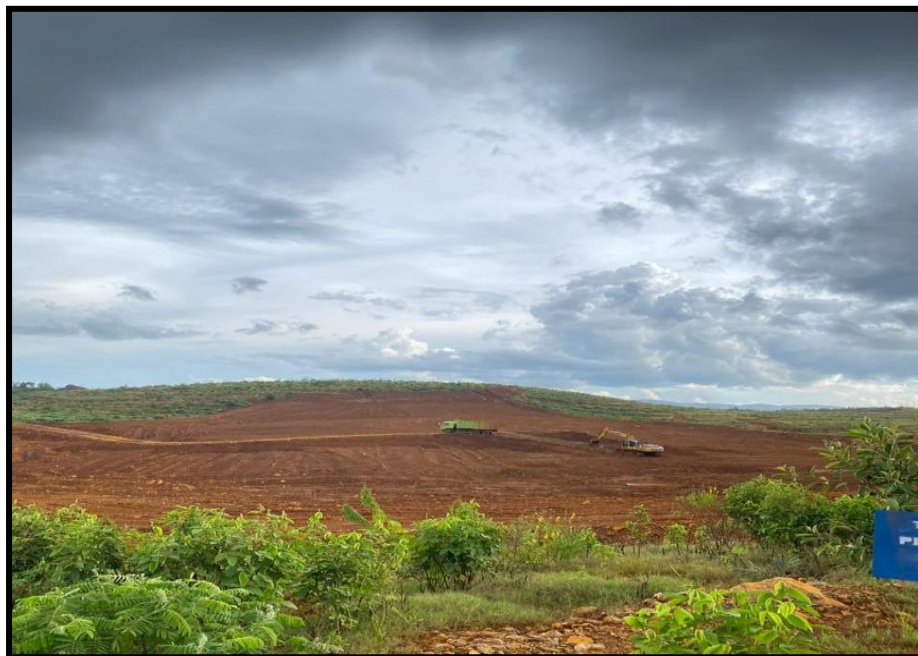
Figure 7 Reclaimed road construction using quarry materials
