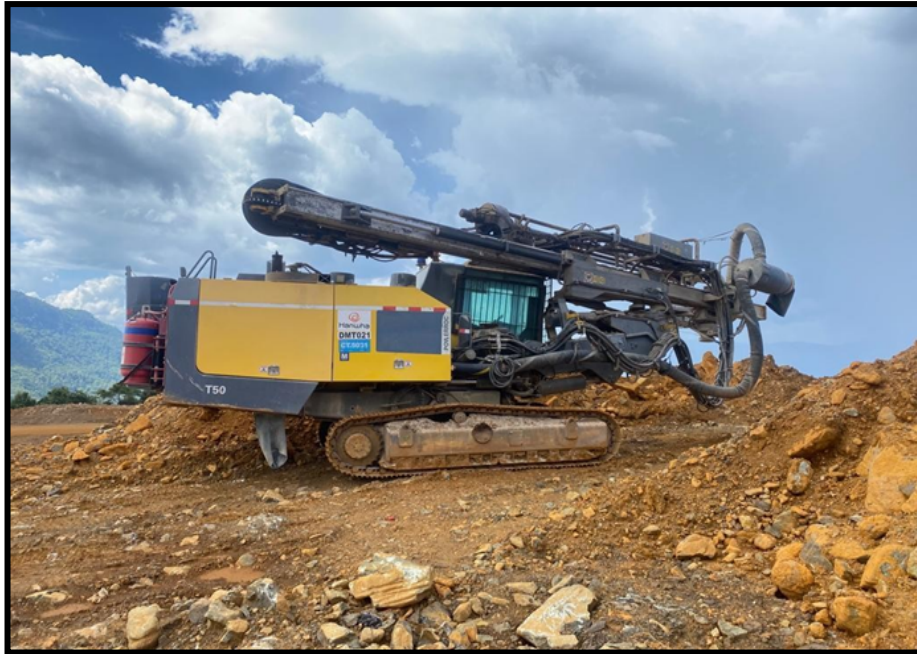
Figure 5 Land levelling process using epiroc T50 heavy equipment
