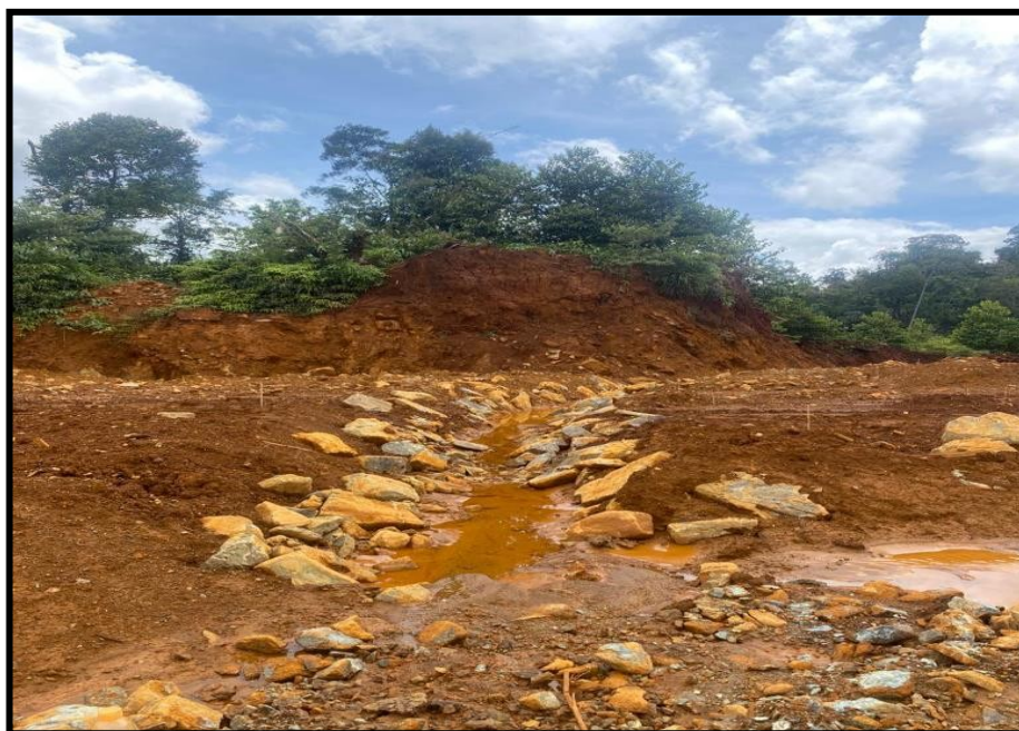
Figure 8 Actual photo of drainage on the Central Pinnacle roundel
