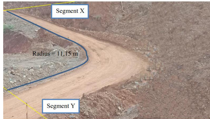
Figure 3. Actual bend radius conditions
