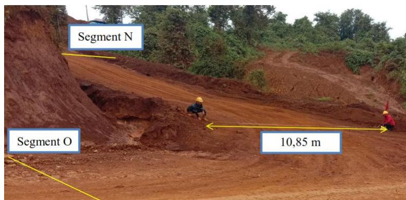
Figure 2. Actual condition of the width of the road on the bend
