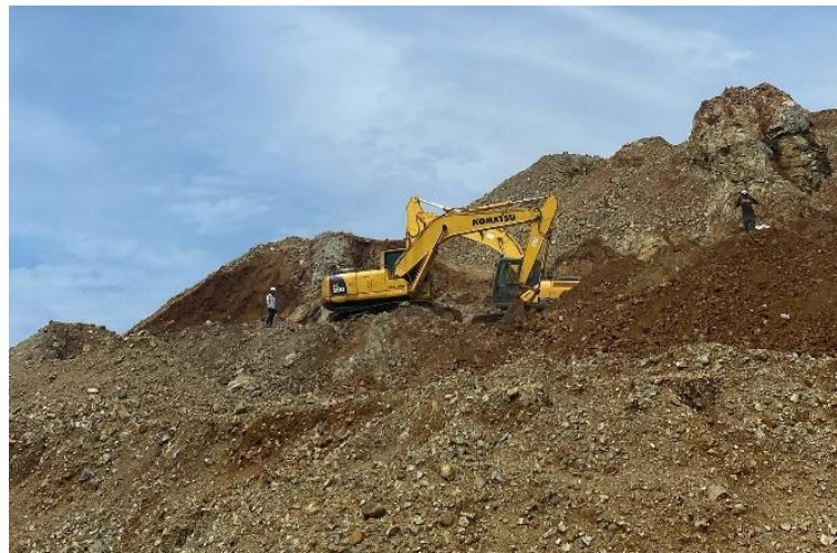
Figure 2. Workers near the Excavator Bucket
